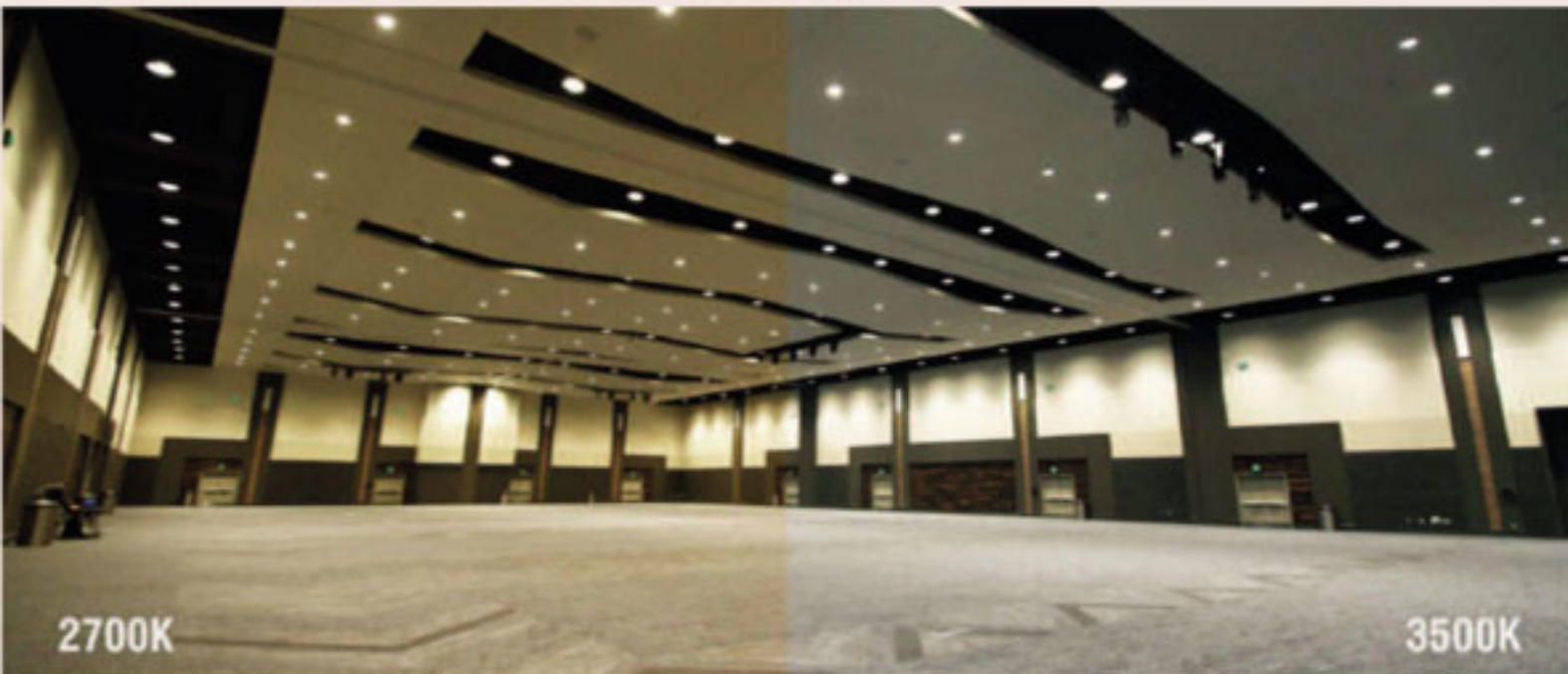
Comparison between the appearances of 2700 K and 3500 K CCT in a convention center
