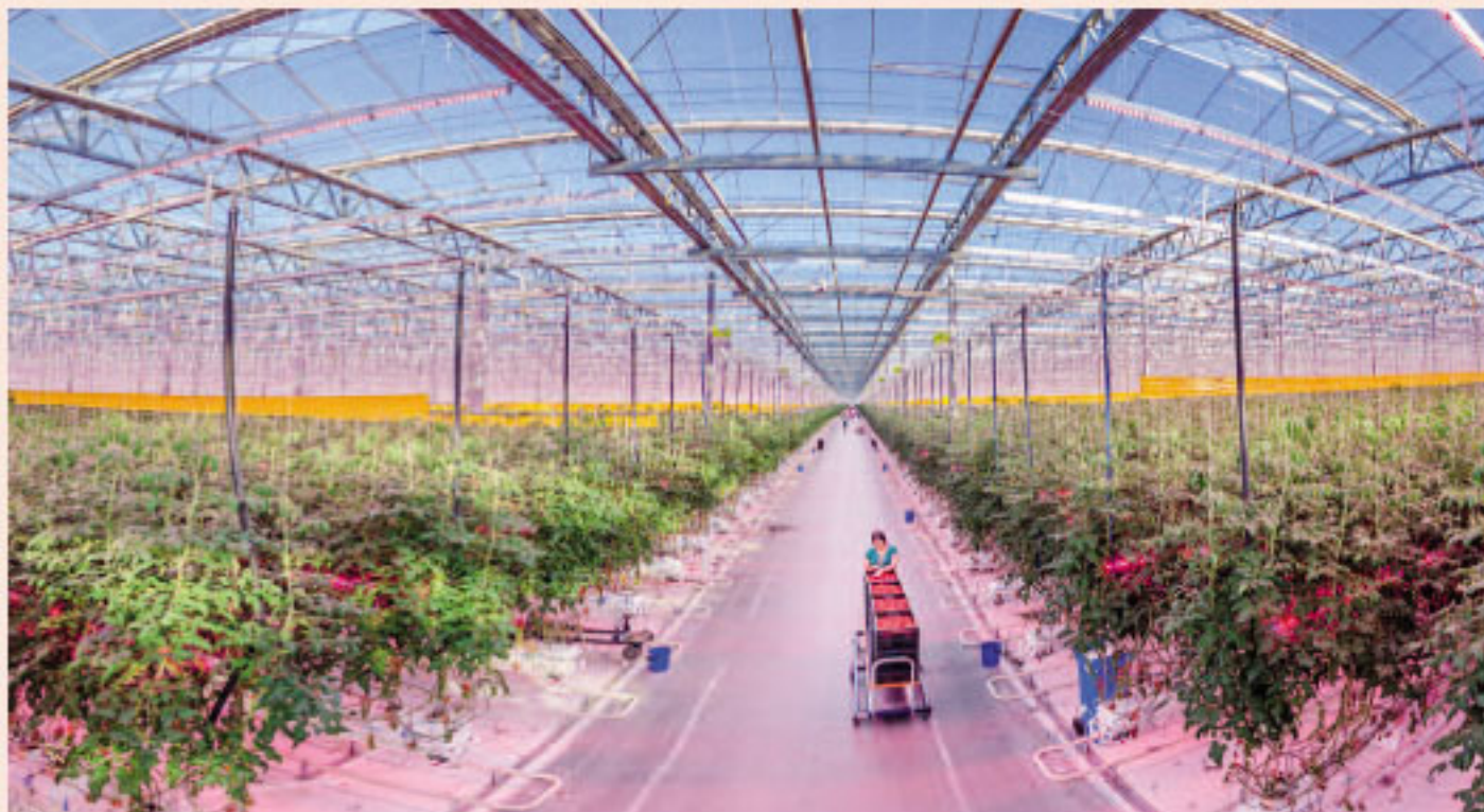
The massive 28-hectare greenhouse – 350 km south west of Moscow, Russia – currently uses over 120,000 luminaires to boost the growth of tomatoes and cucumbers.
