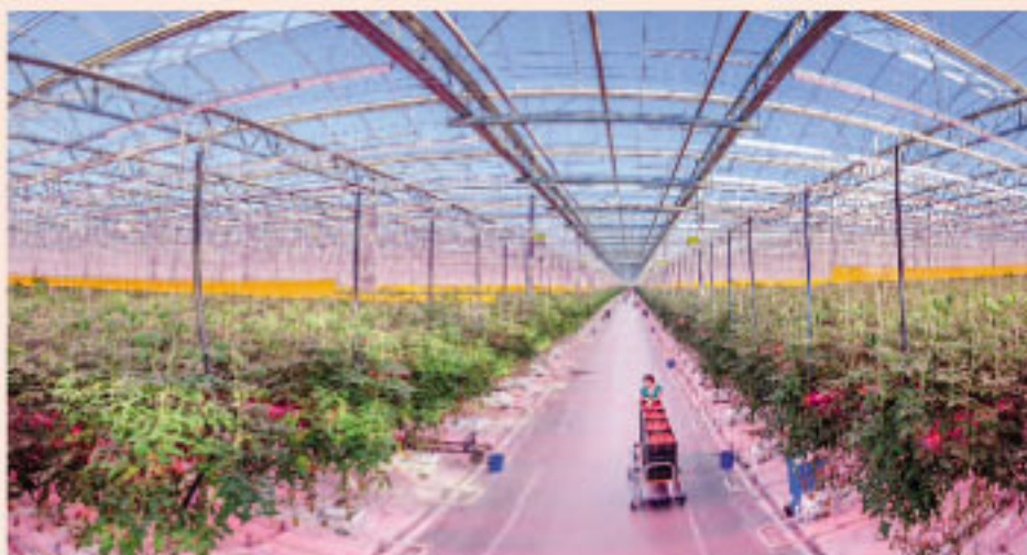
The massive 28-hectare greenhouse – 350 km south west of Moscow, Russia – currently uses over 120,000 luminaires to boost the growth of tomatoes and cucumbers.
