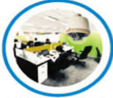
CCTV Kamera Sistemleri CCTV Camera Systems
